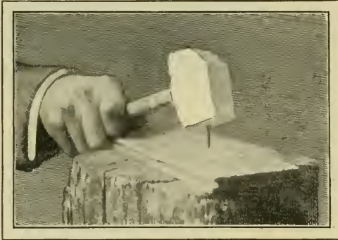
DRIVING A NAIL WITH A HAMMER MADE OF FROZEN MERCURY.
